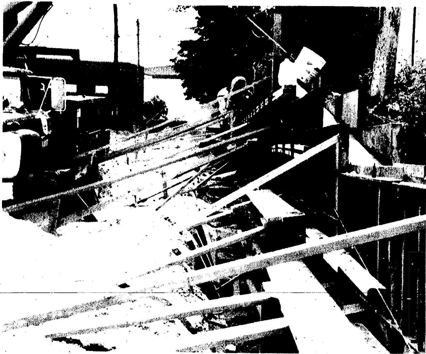
PLENTY OF SUPPORT was provided for a concrete retaining wall being constructed on the western edge of the new downtown Chelsea parking lot between South and W. Middle Sts. The lot is scheduled to be paved either late this week or early next week. It will provide 30 parking spaces.
